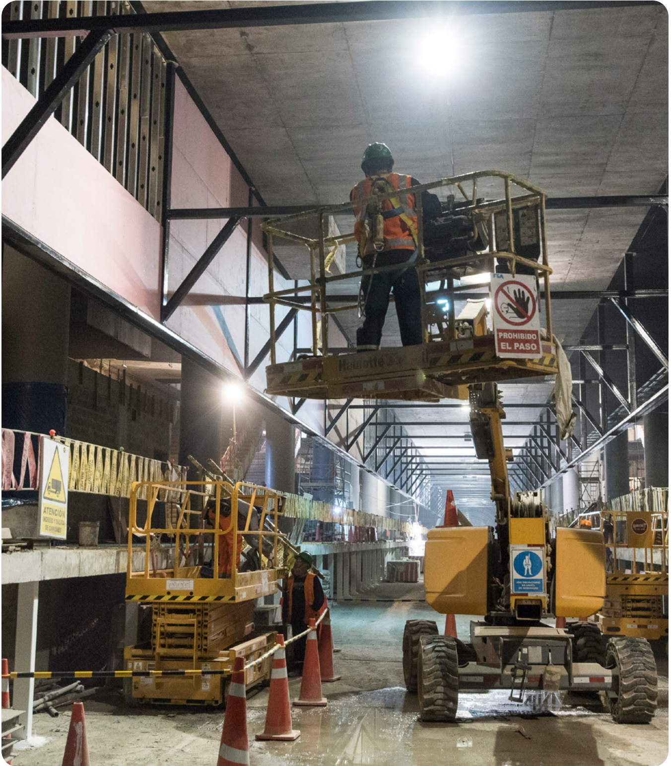
Lima Metro Line 2 station under construction. Photo: Yayo López/World Bank
