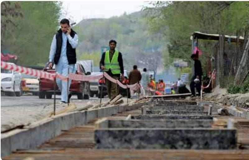
Road construction: median upgrading, side drainage works and culverts. Kabul Urban Transport Efficiency Improvement Project. Makroyan, Kabul, Afghanistan
