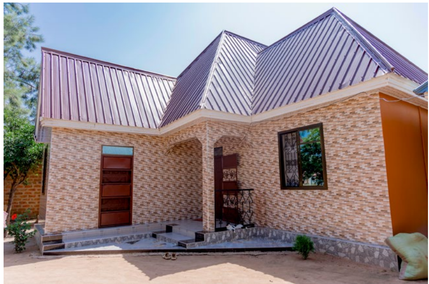
New housing construction near Lake Victoria, Tanzania. Photo © IFC
