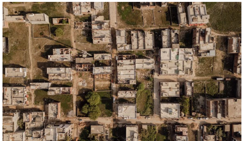
Overhead view of housing in Lucknow, Uttar Pradesh, India. IFC, with FIAS support, is working on initiatives to finance and develop more affordable and energy efficient housing. Photo © JDOT Productions
