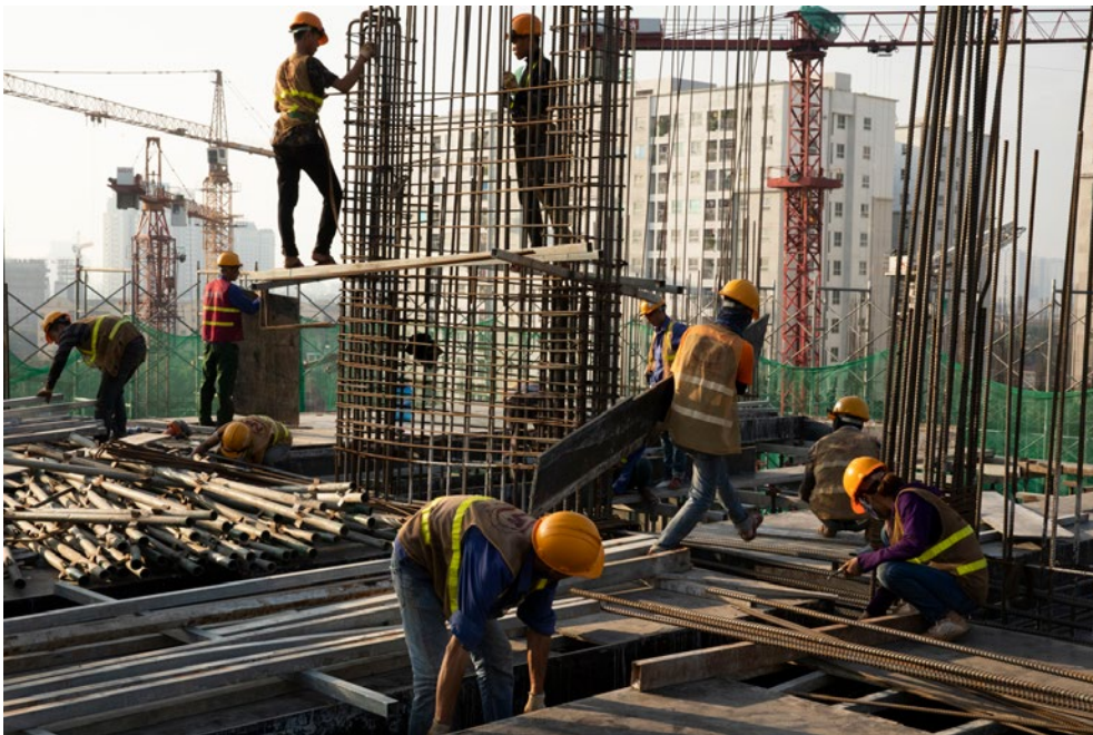
EDGE-certified construction, Hanoi, Viet Nam. Photo: © Dominick Chavez / IFC
