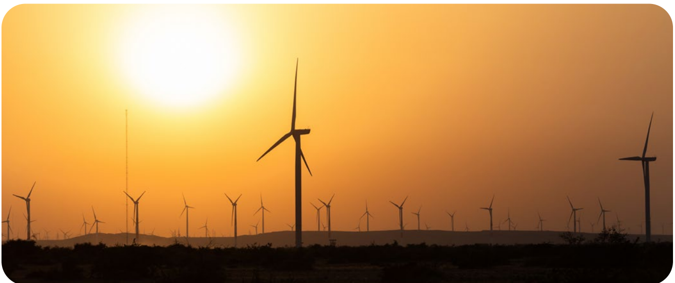
Wind turbines in Jhimpir, Thatta, Pakistan. Photo: © Khaula Jamil/IFC
